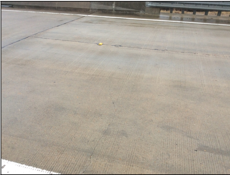
Typical approach slab cracks.
