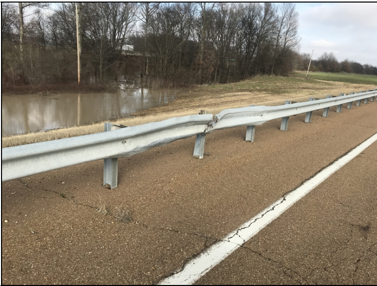
Abutment 2 left approach rail damage 60' from bridge end.
